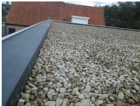
Foto dakplatform in EPDM ter illustratie
