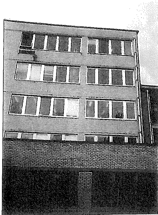
View from internal patios.
