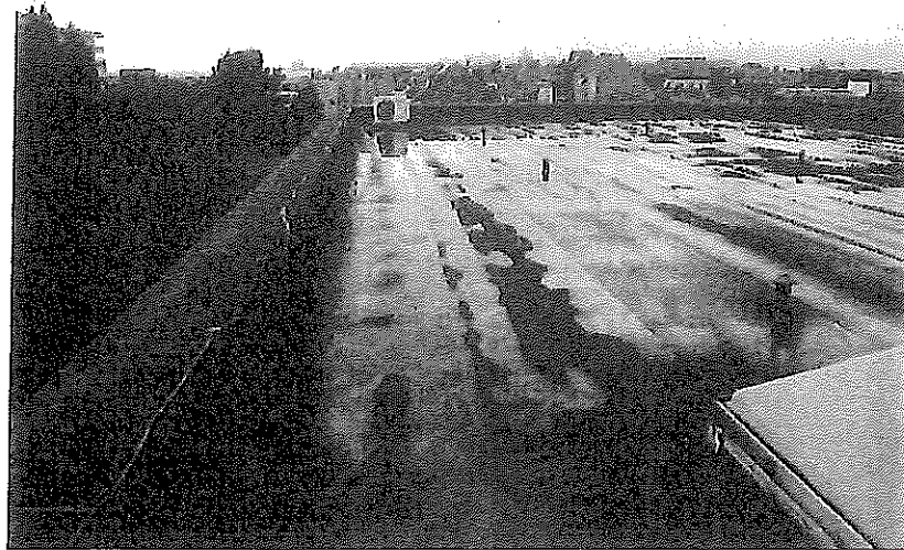
View of roof, office building.
