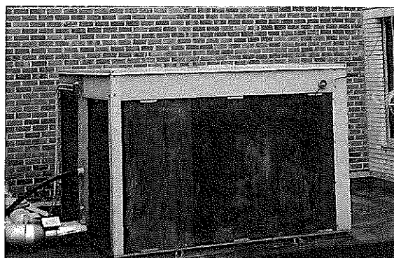
Figure 7 : Existing cooling machine (Trane® monobloc chiller with scroll compressors)
