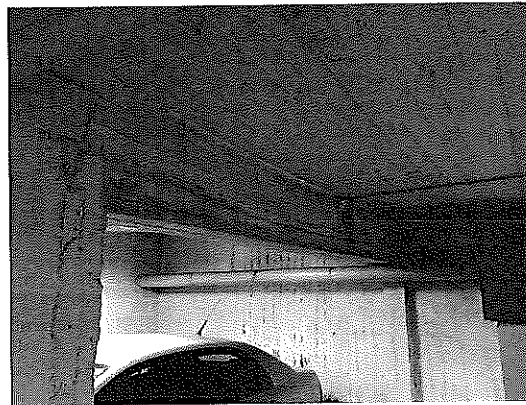
Figure 2 : Deformation of the slab
