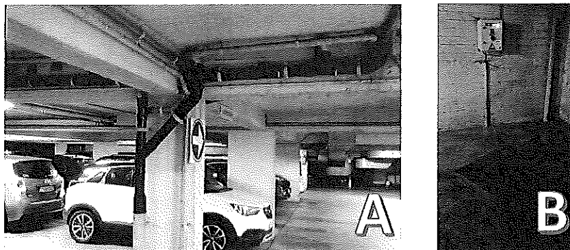
Figure 10 : Sewage system – (A) HDPE (black) and PVC (white) pipes; (B) Location of the wastewater pump
